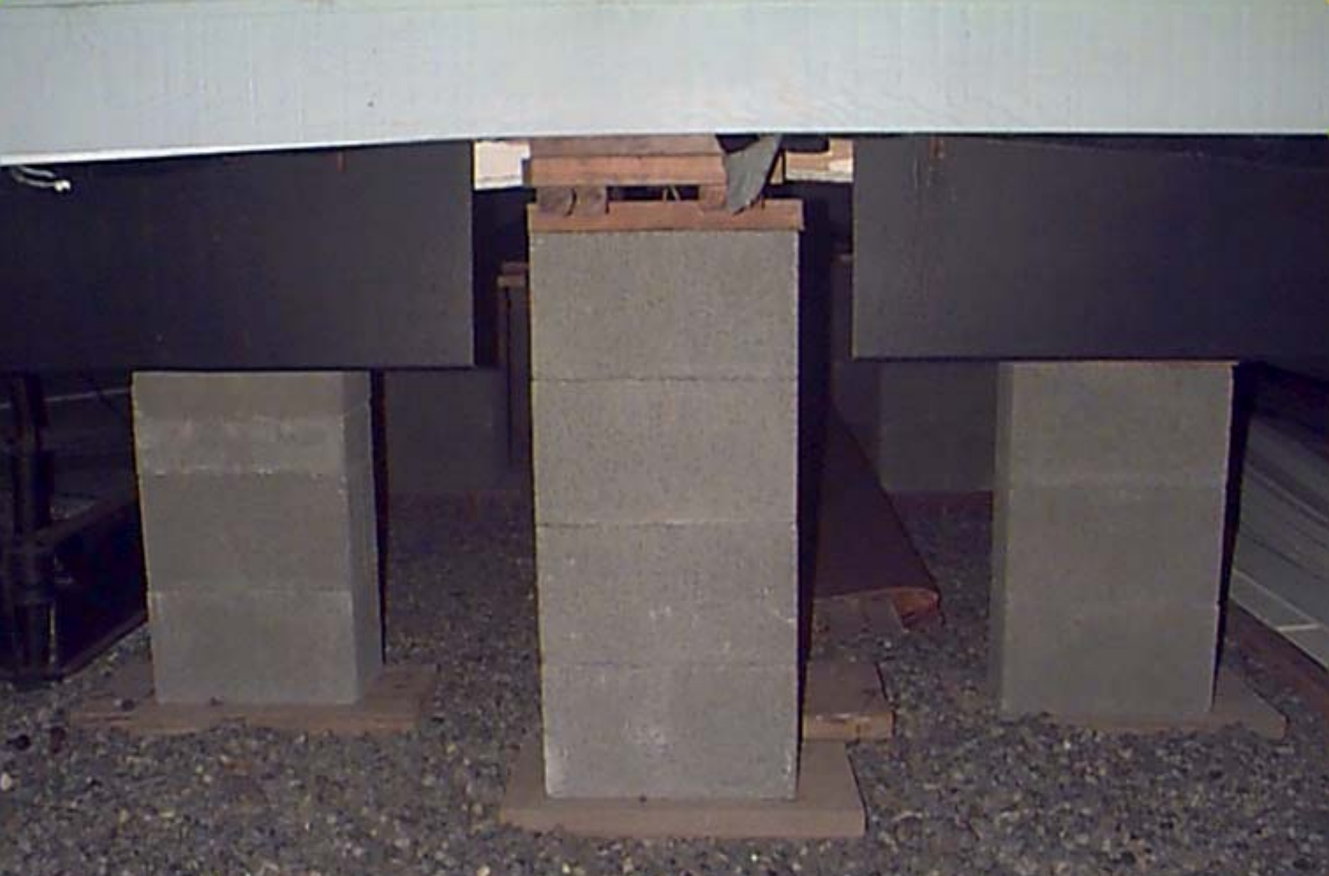
Properly erected piers on proper footings
