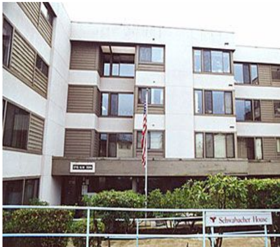
Schwabacher House will receive extensive exterior repairs in 2008.
