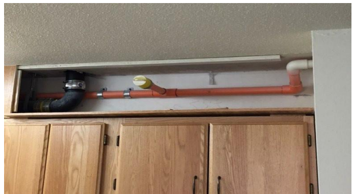
New Fire Sprinklers in an MPHA Unit
