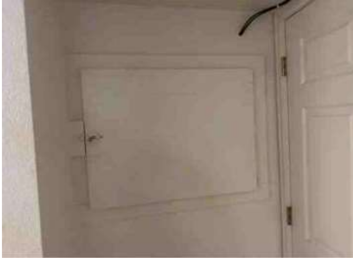
Crawl Space Access
