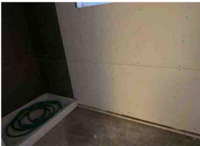
Basement - Roughed in Bath
