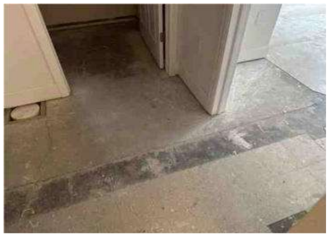
Basement - concrete flooring
