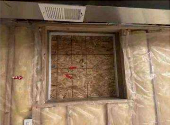
Crawl Space Access
