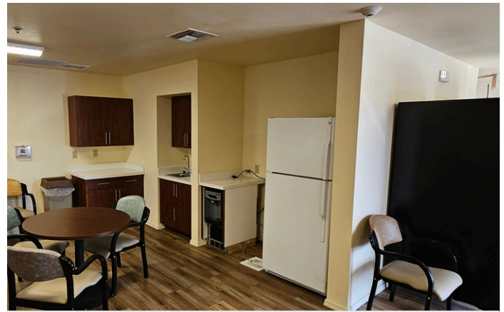
Renovated community room
