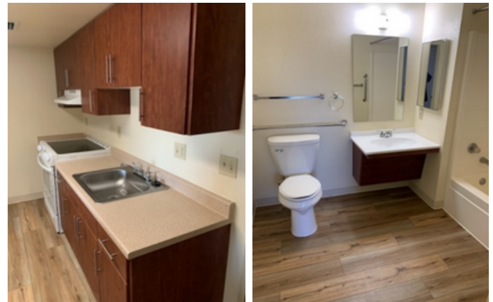
Residents love the new in-unit kitchen and accessible bathrooms with grab bars.
