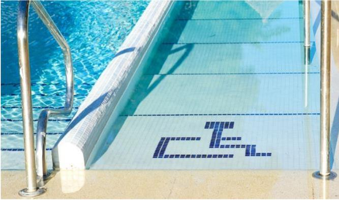
Access to swimming pools includes the ability to enter and use the pool deck area and the ability to enter and use the pool. Access to the pool deck should be via an accessible path and an accessible gate. Modifications to pool entrance equipment may include ramps, permanent and portable lifts, and platforms. Guidance in the new ADAAG Standards for swimming pool access is found at ADA Accessibility Standards at [Access-board.gov](http://Access-board.gov).
