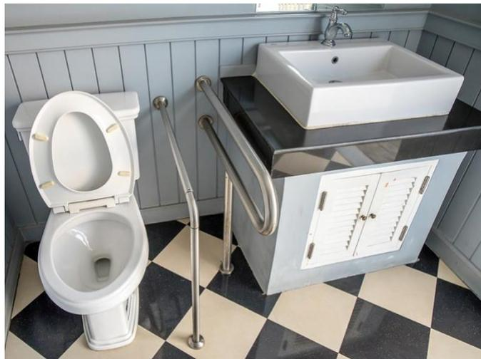
The most often cited example of a reasonable modification is the installation of grab bars at the toilet, tub, or shower. Because the Act's design and construction requirements only address the installation of reinforcements in walls for later installation of grab bars, the addition of grab bars is a modification that may be requested both in recently constructed and older housing.
